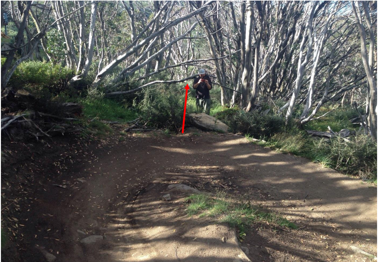
Photo 1: This existing corner which is too tight will be removed and rehabilitated with the trail alignment heading through the trees to the north as shown in red.
