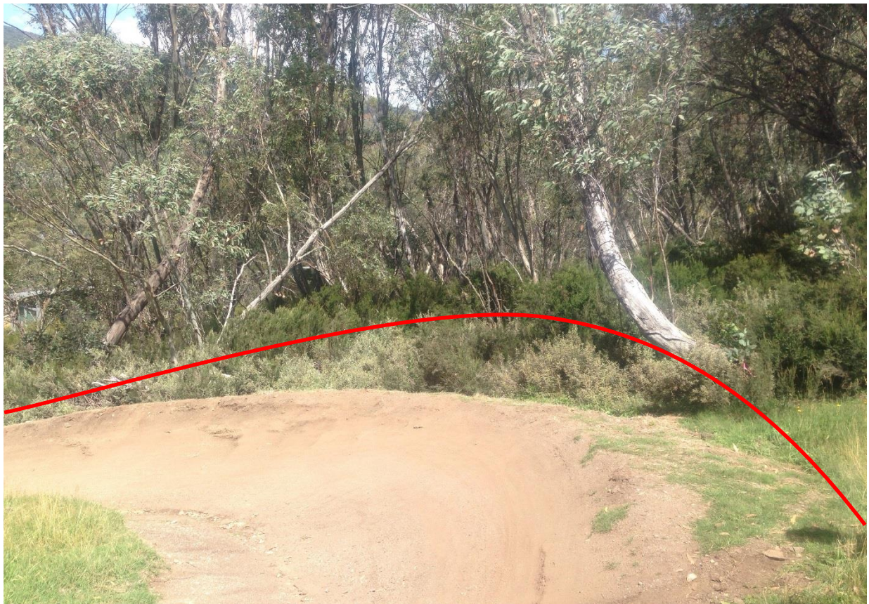
Photo 16: Section 7 involves extending the corner further into the regrowth subalpine woodland so that the corner is off the ski run.
