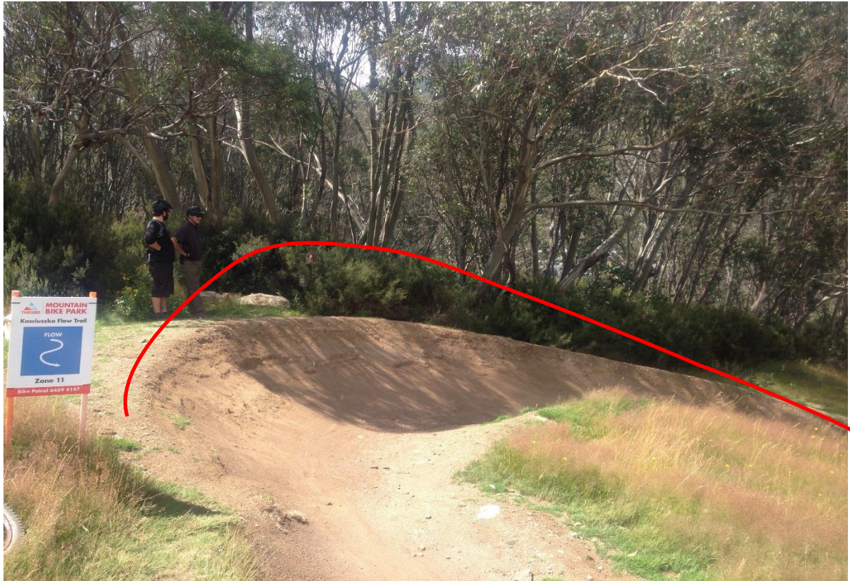
Photo 15: Section 6 involves extending the corner further into the regrowth subalpine woodland tree island so that the corner is off the ski run.
